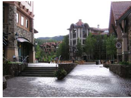
Figure 23. Telluride, Colorado. Gateways can be formed by constricting buildings before opening into a wider space.
